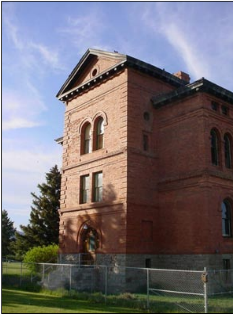
Side view, Asylum Building, Boulder River School, Jim Jenks, photographer, © 2005 Jim Jenks.
