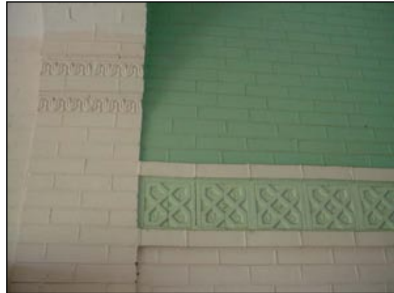
Pressed brick, Asylum Building, Boulder River School, Chere Jiusto, photographer, © 2005 Chere Jiusto.
