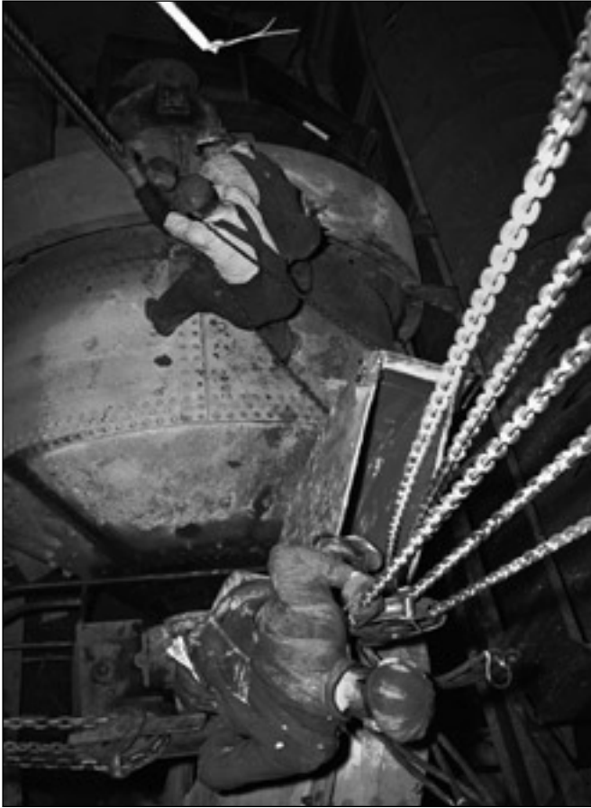
Lowering new machinery, Flotation, Washoe Smelter, Anaconda, 1942. Photograph by R. I. Nesmith. Courtesy Montana Historical Society Research Center Photograph Archives, Helena (Lot 19 A102).
